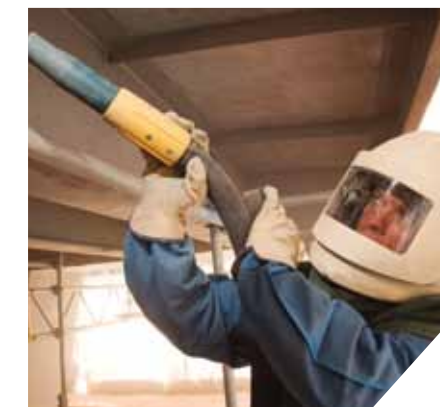
Sandblasting on the CBH Shiploader Refurbishment Project, Kwinana, Western Australia
