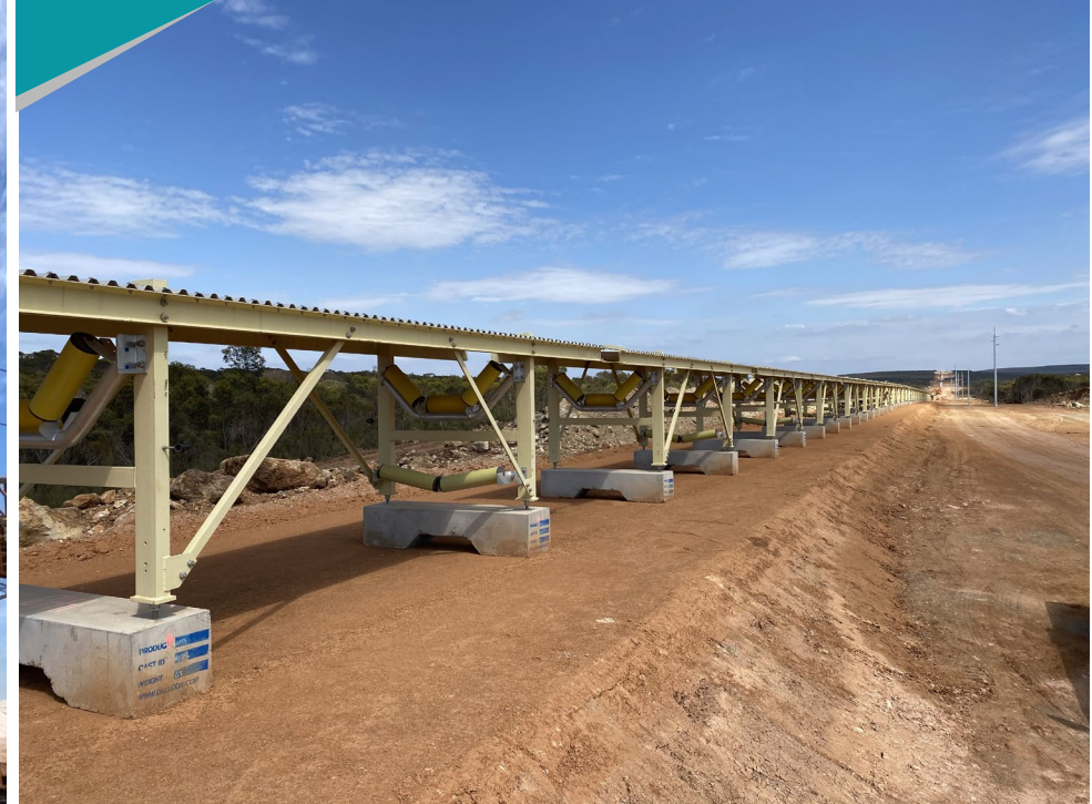
AusGroup installing a 9km overland conveyor at First Quantum's Nickel mine in Western Australia
