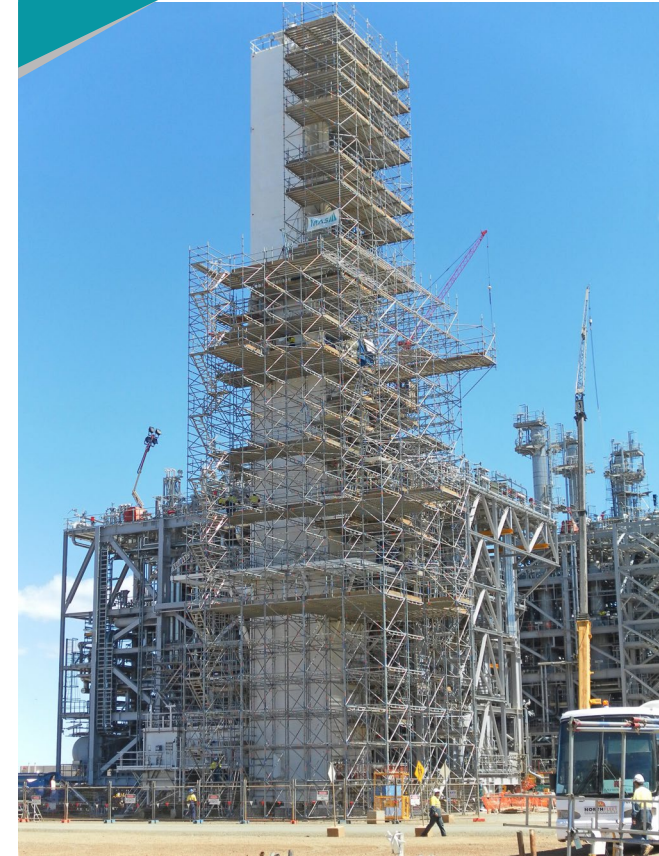
AusGroup – MAS scaffold erection at an LNG facility
