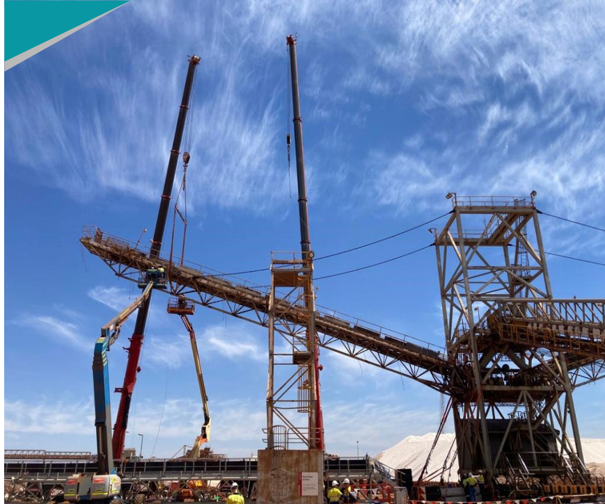
AusGroup completed the fabrication and installation of the twin boom stacker work at the Rio Tinto Dampier Salt
