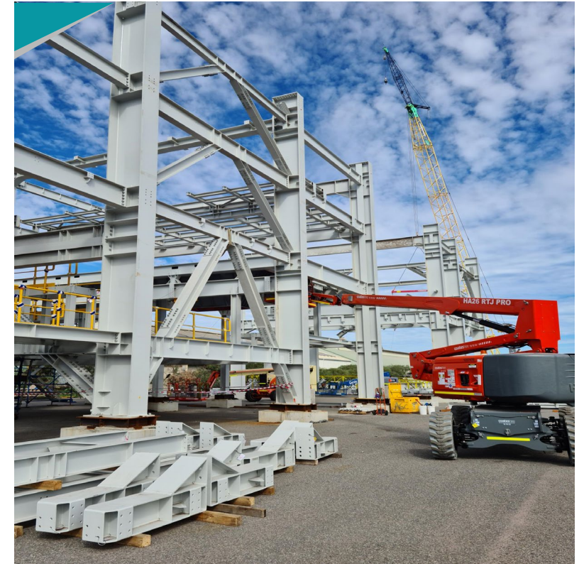
AusGroup fabricated, assembled and delivered Waste to Energy modules
